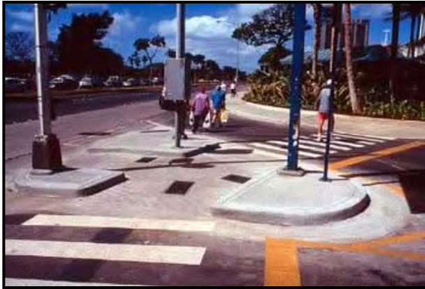
Exhibit 6-8: Pork Chop Island with textured surface and ADA compliant curb cuts
