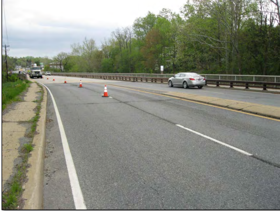
Route 2 (Kirkwood Highway) – East of Newark
