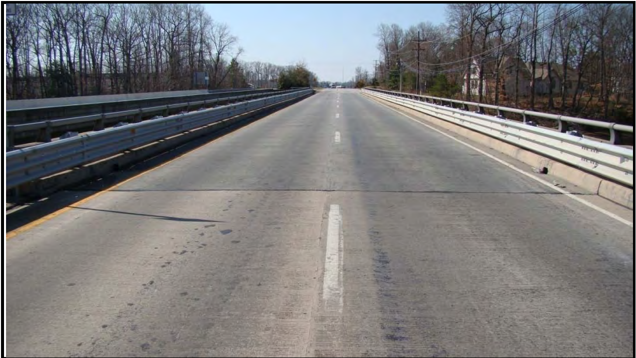
Route 10 over St. Jones River – Looking West
