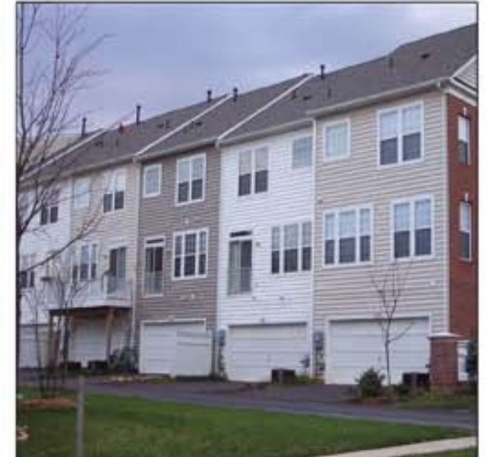
Townhouse Units with Alley Access Gaithersburg, Md.
