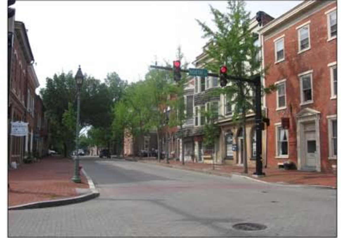
Existing Building Context State and North Street
