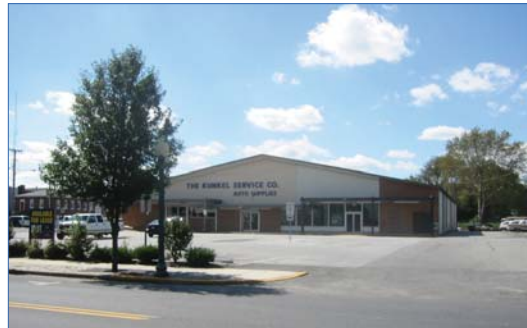
Figure 3-1: Wide Curb Cuts: Contributor to Negative Pedestrian Perceptions
