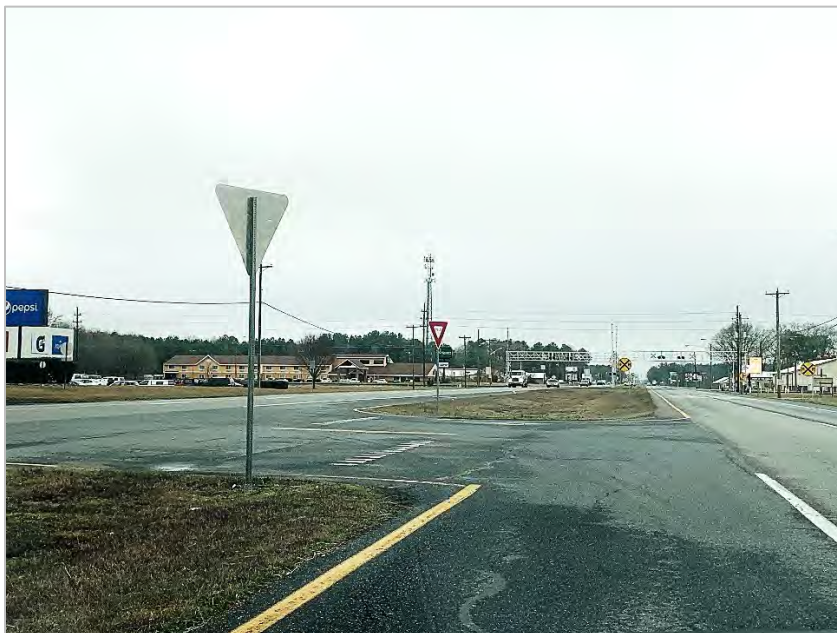
US 13 median at Clukey Drive. The DCR grade crossing of US 13 is seen just to the south.
