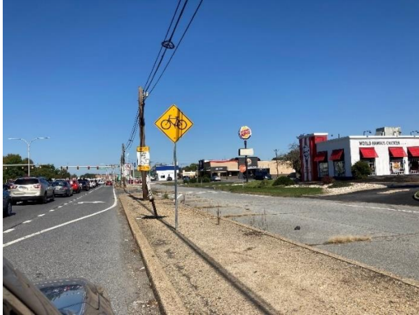
Figure 1 (l): US13 northbound, next to KFC and Burger King. The elevated curbs in front of these properties are not suitable for use as sidewalks.
