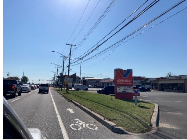
Figure 1 (l): US13 northbound, next to KFC and Burger King. The elevated curbs in front of these properties are not suitable for use as sidewalks.
