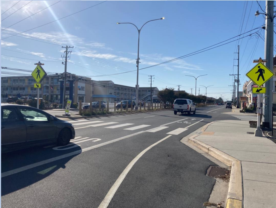
Rapid Flash Beacon (RFB) and midblock crossing (Example from Dewey Beach)
