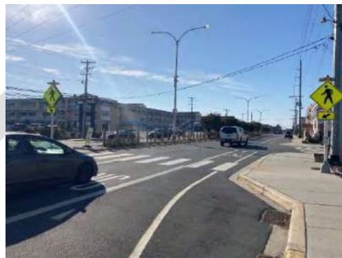
Figure 24: A Rapid Flashing Beacon (RRFB) and pedestrian refuge island in Dewey Beach.
