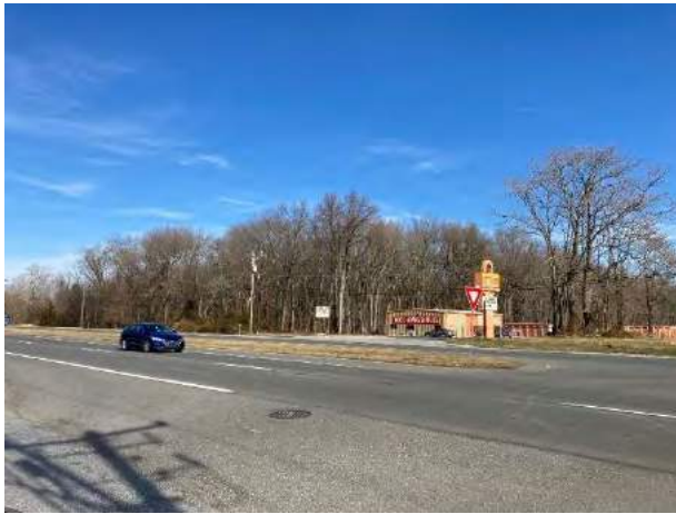
Figure 20: The existing Pinewood Acres intersection, which does not have a traffic signal.
