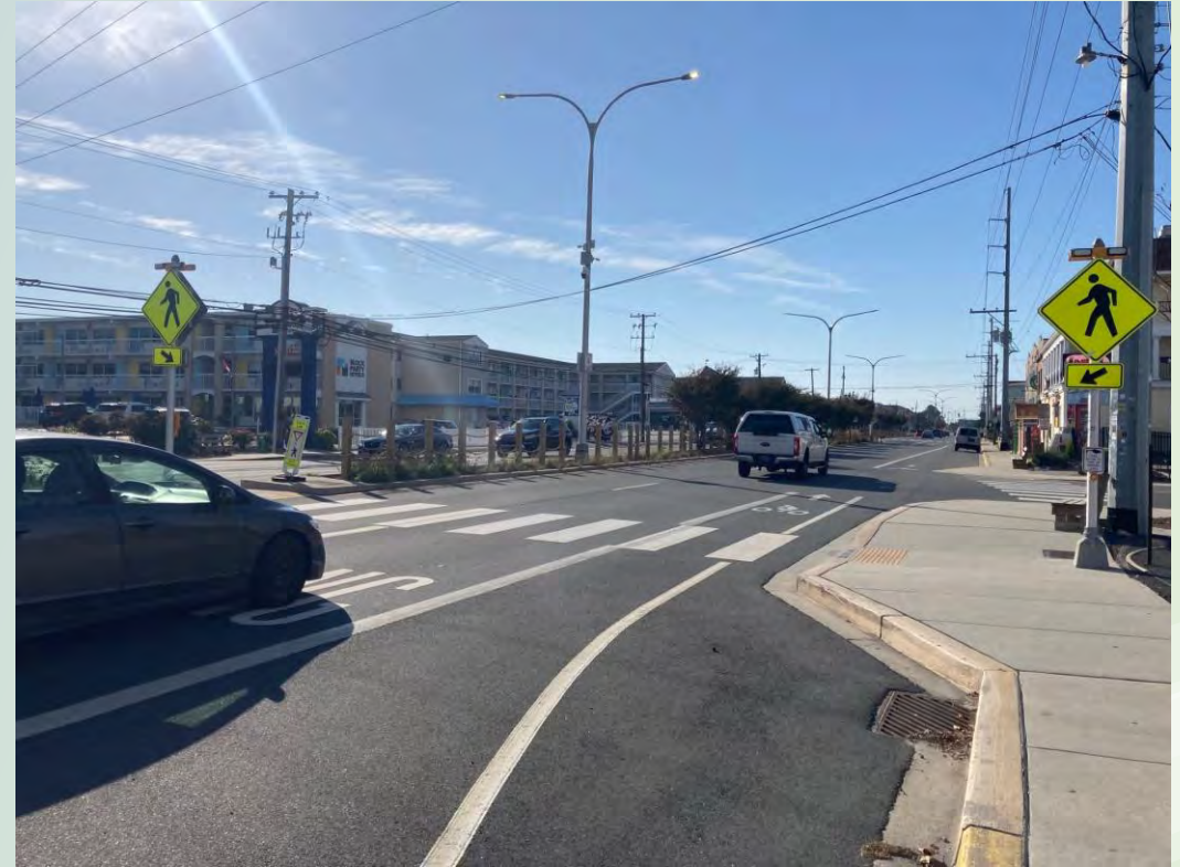
Rapid Flash Beacon (RFB) and midblock crossing (Not appropriate for conditions of US13)
