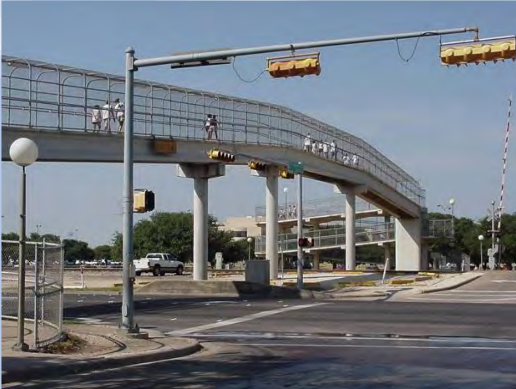
Pedestrian bridge over US13 (Not cost-effective or conducive to pedestrian safety)
