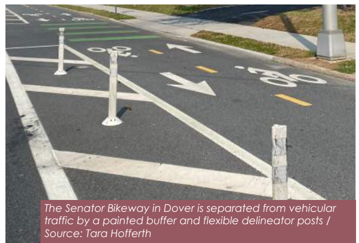
Bike lane separated from traffic by flexible delineator posts and concrete pills / Source: Aditya Inamdar
