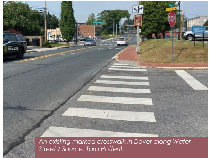
Wide high-visibility crosswalk markings at a high volume intersection
