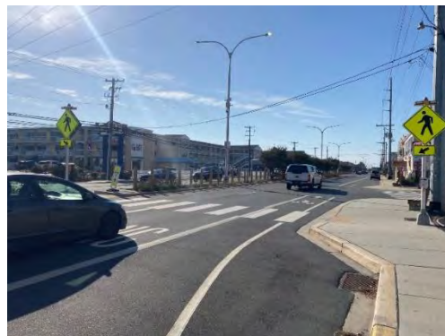
Figure 27: A Rapid Flashing Beacon (RRFB) and pedestrian refuge island in Dewey Beach.
