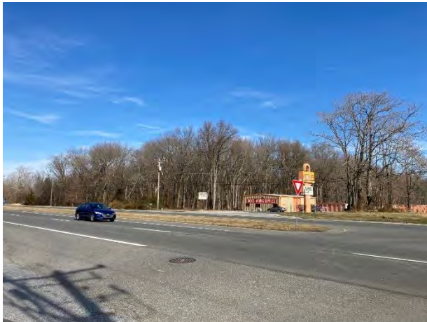
Figure 23: The existing Pinewood Acres intersection, which does not have a traffic signal.
