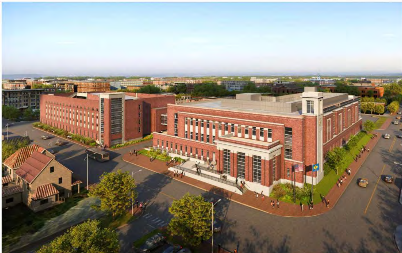
AERIAL VIEW – GOVERNORS AVENUE. & WATER ST.
