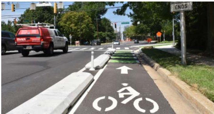
Bike lane separated from traffic by flexible delineator posts and concrete pills / Source: Aditya Inamdar
