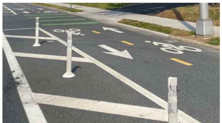
The Senator Bikeway in Dover is separated from vehicular traffic by a painted buffer and flexible delineator posts / Source: Tara Hofferth
