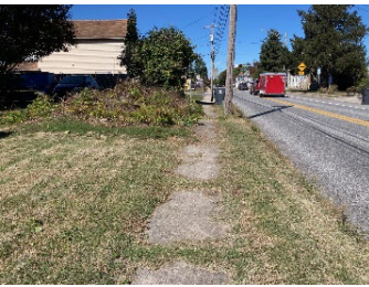
Repair existing sidewalks
