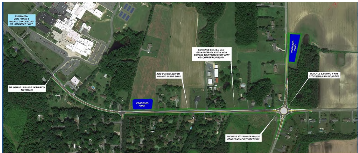
Figure 13: Walnut Shade Road Project
