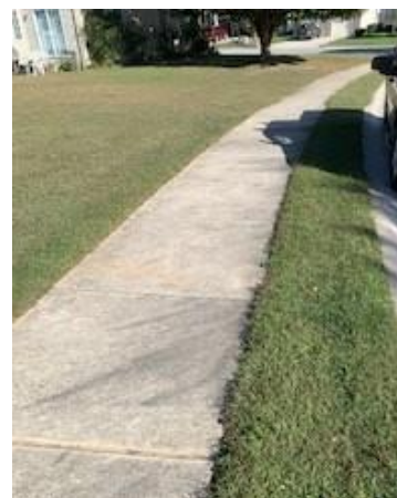
Figure 7 Typical 5 Foot Sidewalk in the Pharsalia Neighborhood as per Camden Code
