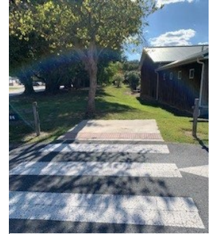
Figure 6: Shared-Use Path Terminus at Brecknock Park
