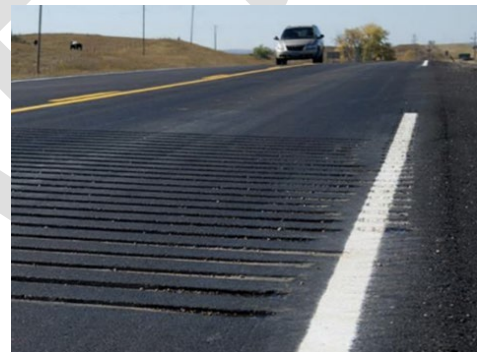
Figure 23: Transverse rumble strips positioned across the travel lane. Source: visionzero.nd.gov ( link ).
