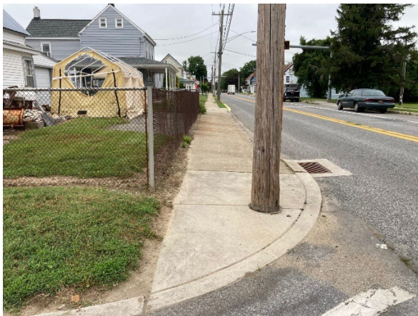
Figure 19. (l): A utility pole obstruction at the corner of Main Street and Wilson Lane.
