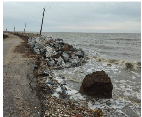
Figure 15: Coastal erosion of Port Mahon Road. Source: Dover Air Force Base – Compatible Use Plan.
