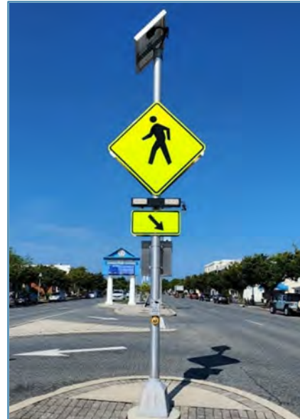
Figure 41: RRFB at Rehoboth Beach, Delaware
